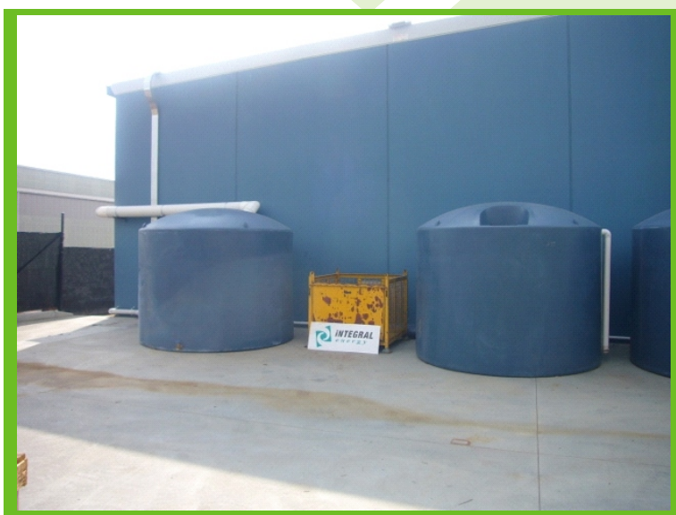
Rainwater Harvesting and Water Filtration/Sterilisation Systems
